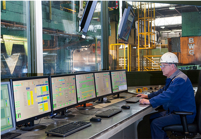
Reference: V7 Control room
